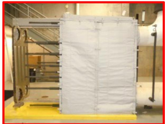
Custom fabricated removable insulation systems provide personnel protection, heat loss & heat gain protection, freeze protection. For heat loss and heat gain, energy savings payback is typically measured in months.
